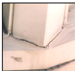
Sealant Separation
