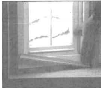
7-c: Install Interior Window Stops
