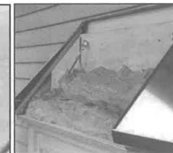
Insulate all Roof Cavities
