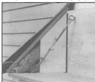
Complete Turn Buckle Hanging System
