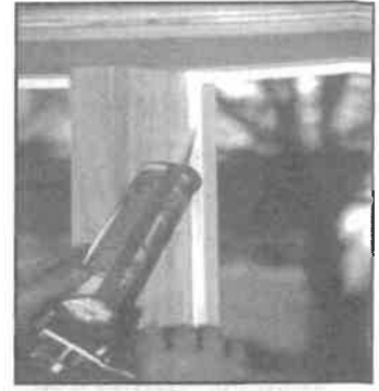
7-b: Insulate between Windows and Frame
