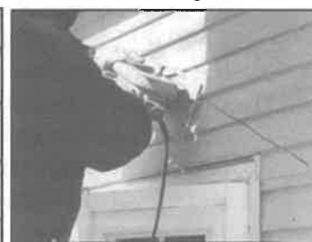
Install J-Channel over siding edge
