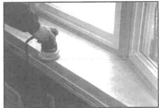
Lightly Sand all Interior Wood Surfaces
