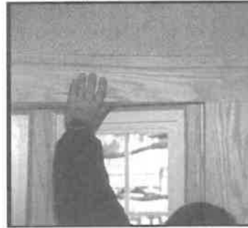
Lightly Sand all Interior Wood Surfaces
