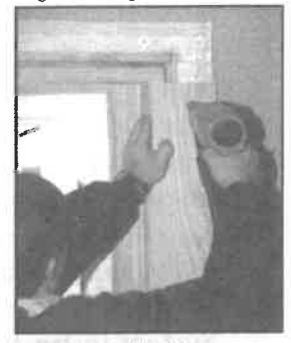
10-i: Fasten 2-1/4" casing to perimeter
