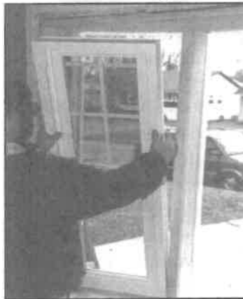
7-c: Install Interior Window Stops
