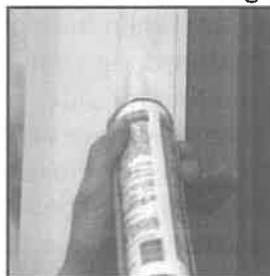
Seal Exterior of Window Units to Frame Window Stops
