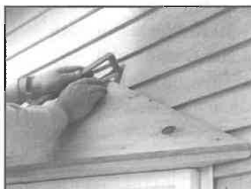
Position Roof Centered on Frame
